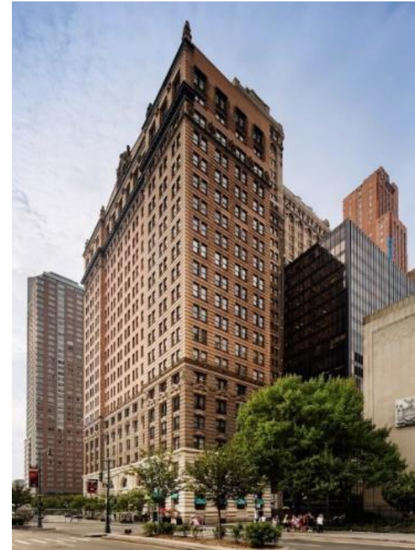
17 Battery Place-South Tower New York, NY
