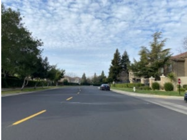
View north on East Taron Road
